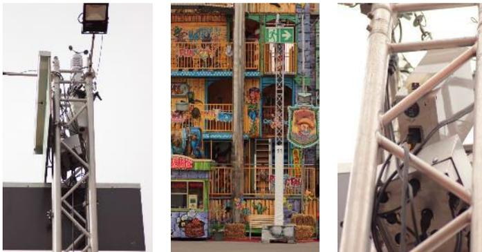
**Figure 23: Deployment of environmental sensors with wind speed meter**
